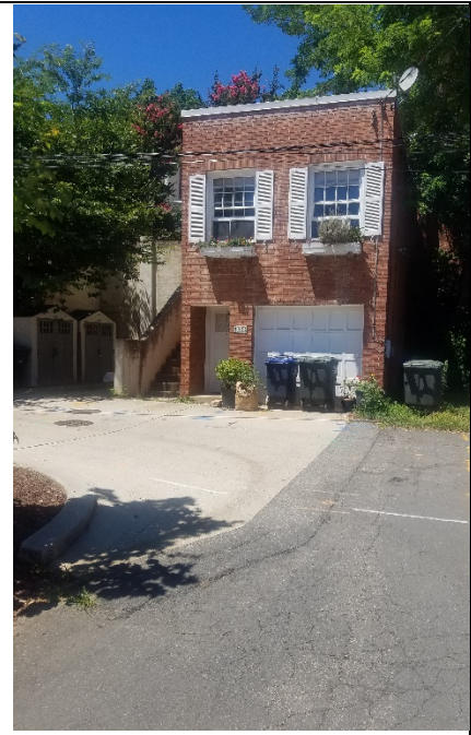
1912 Whitehaven Parkway (alley facing 36th St; apparent second-story living space)
